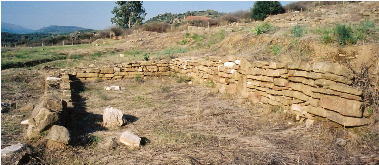
Fig. 103. Stratos, 'Byzantine building 1', view of the E inner façade.
